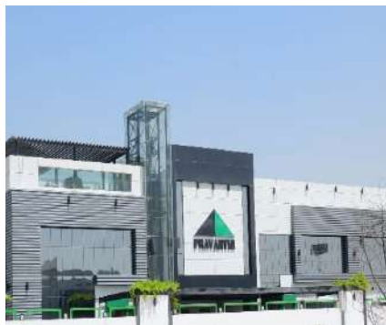
PRAVARTHI FIRE | Jebel Ali Free Zone
